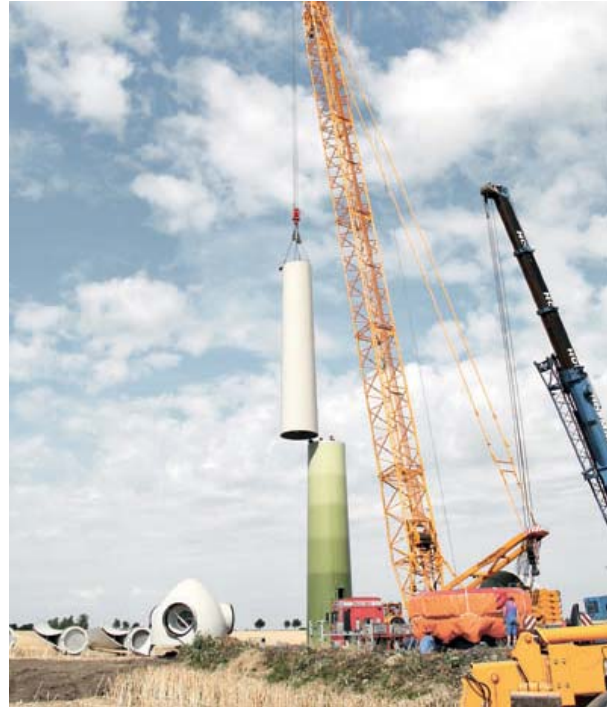
The tower segments are installed using a special crane.
